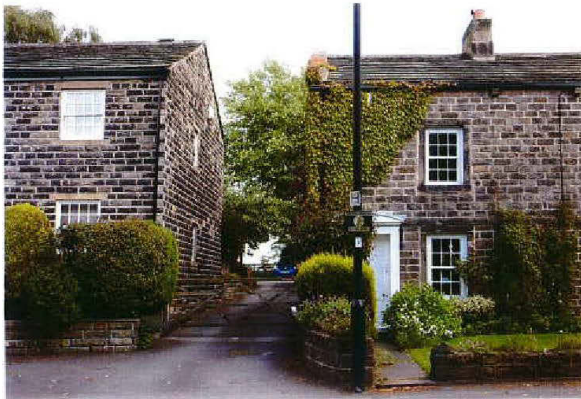
Plate 9 View of one of the gaps between listed terraces on Main Street looking east towards the currently open land to the rear
