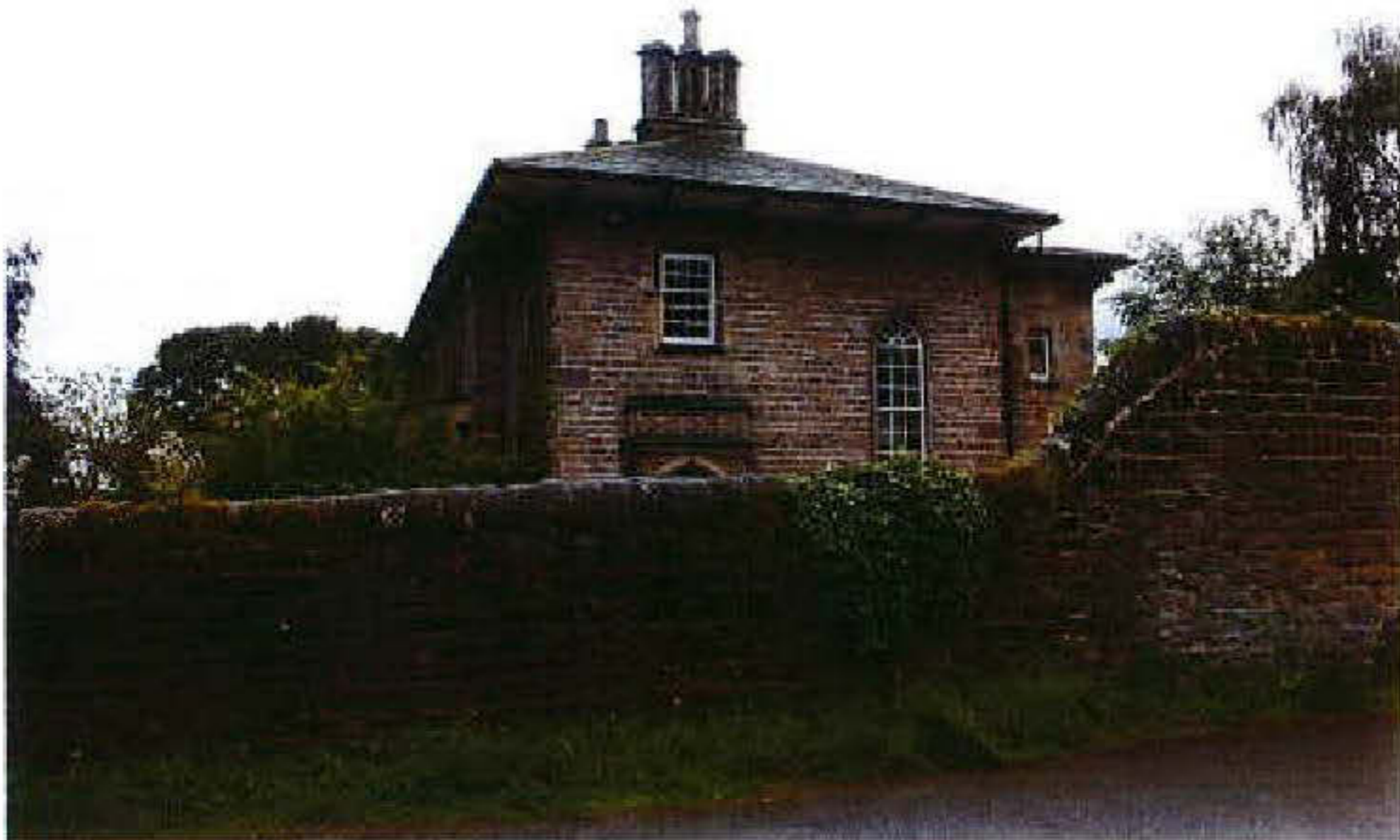
Plate 6: View of Burley Hall and part of its separately listed stone garden wall looking south
