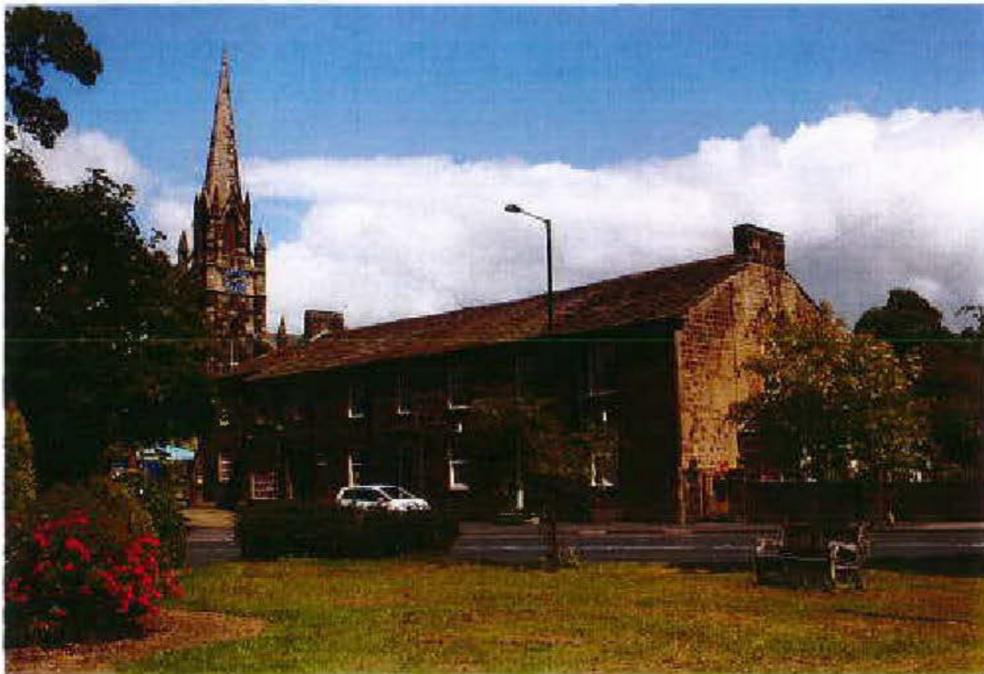
Plate 5: View of the terrace of stone cottages at 24-30 (even) Main Street incorporating No 2 Post Office Yard. Note the Parish Church of St Mary in the background
